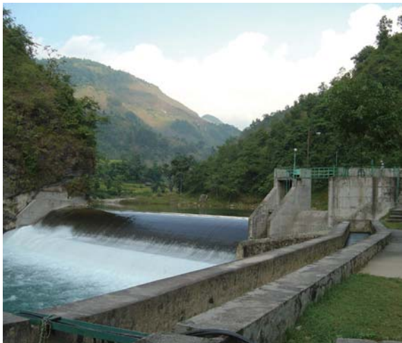
<Picture 2> Intake and the Settling Basin
