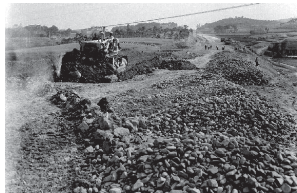
<Access road construction>
