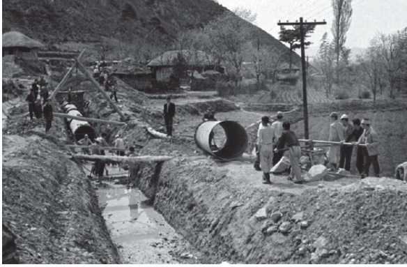
<Industrial water and road construction>
