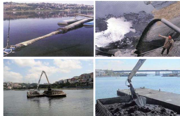
<Picture 7> Sludge dredging in the Golden Horn Estuary
