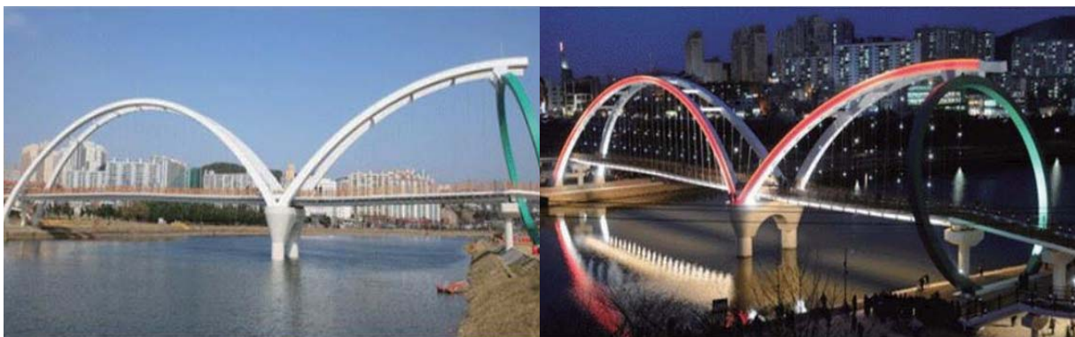
Source: Taehwa River Web site
