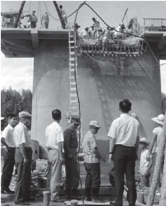
<Intake tower construction>
