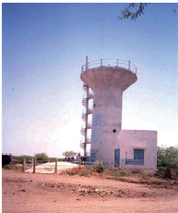
<Picture 3> Elevated Service Reservoir with Pump House in a Village, Saurashtra, Gujarat
