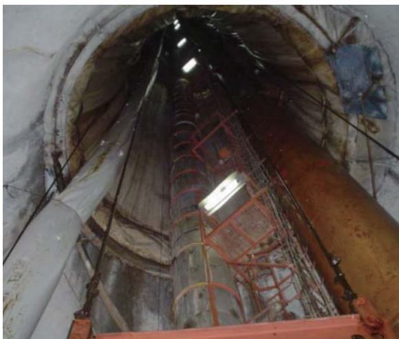
<Picture 3> Drop Shaft for Penstocks
